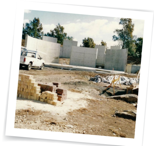
▲ The Memorial Centrepiece under construction in early 1996.
